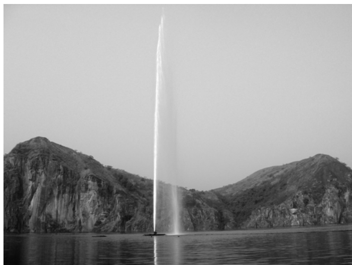
photo 3. Recent degassing fountain and pipe raft at Lake Nyos (Jan. 2006)
